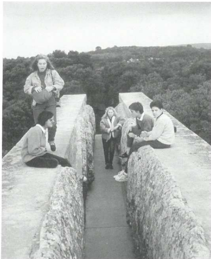
Dried-out 7th grade on a dried-out Roman aqueduct.
